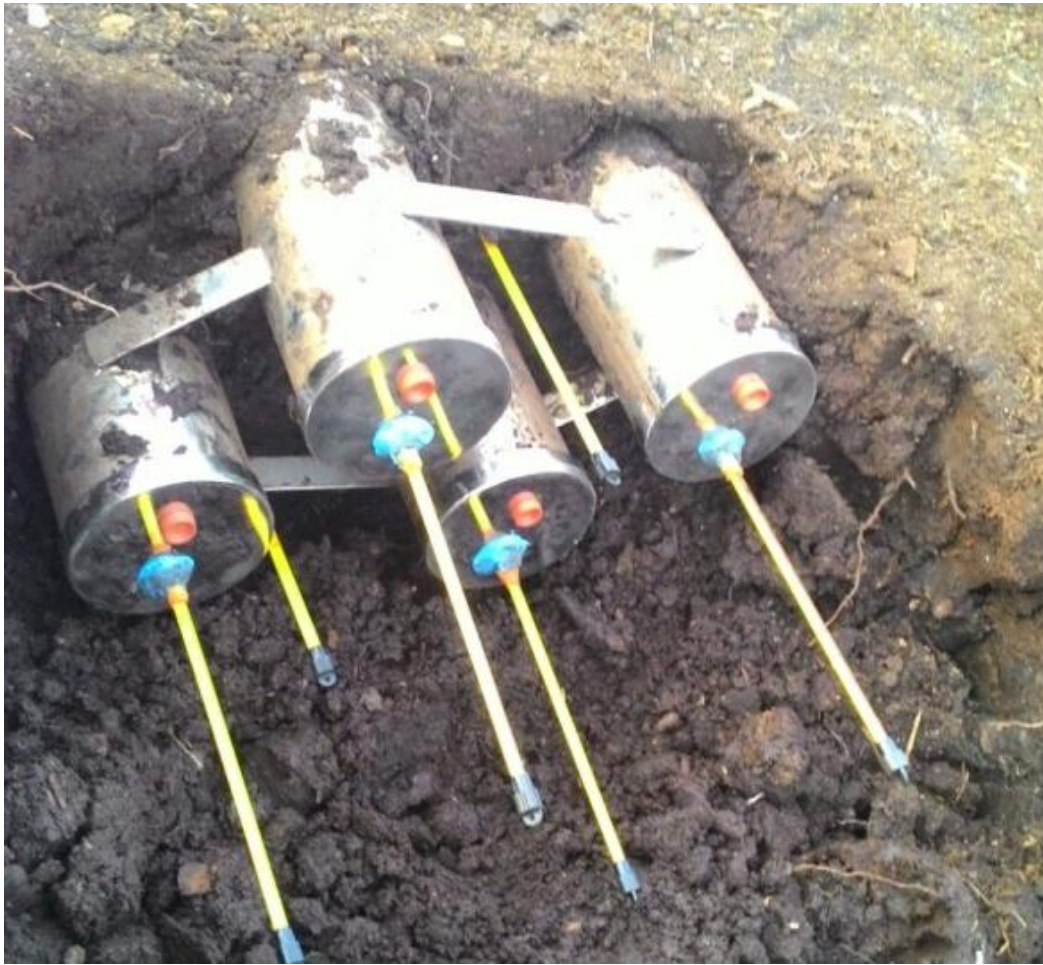
Figure 2. Fabricated L-shaped chamber installed horizontally to the wall of the peat soil pit to a distance of 20 cm
