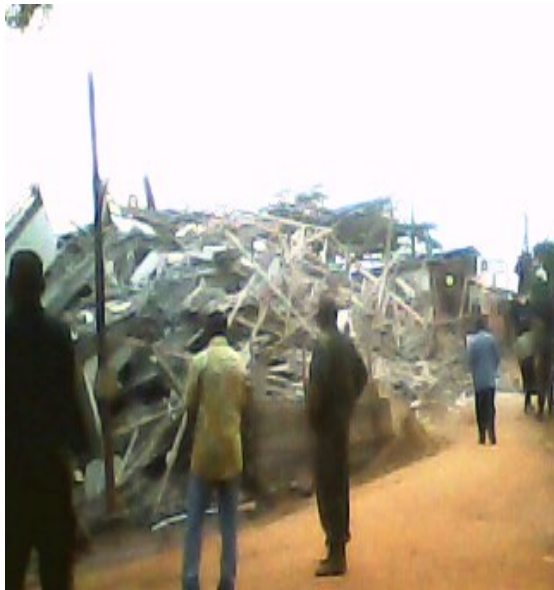
Figure 1. Building collapse at Elig-essono Suburb, Yaoundé
