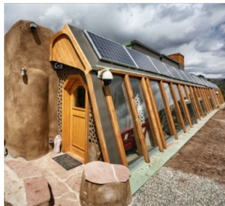
Figure 3. Earthship dwelling, Greater World Community, Taos, New Mexico (2017)
