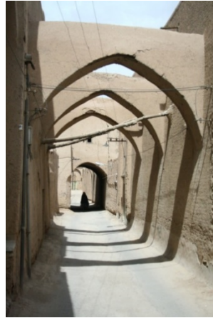
Figure 1. A street in yazd city: Narrow streets with tall walls are used to make more shaded spaces. Moreover some part of the street has been covered to increase these shaded spaces
