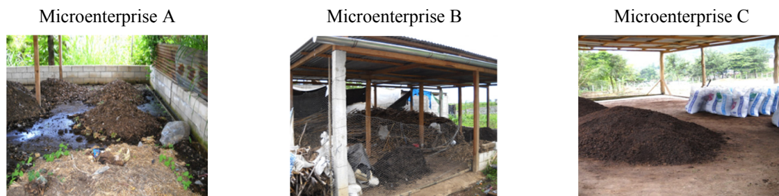
Figure 3. Structures housing compost operations
