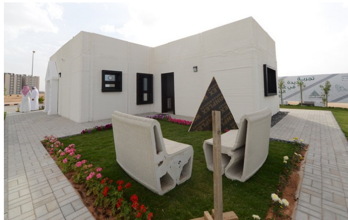
Figure 4. The first house in the Middle East to be built in 25 hours using 3D printing
