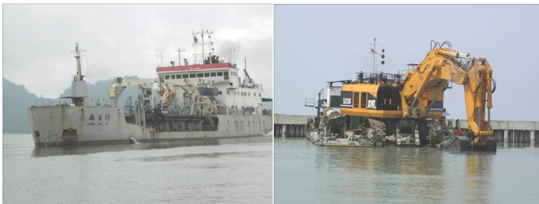
a) Trailing suction hopper dredger (TSHD) (Lumut, Perak)
