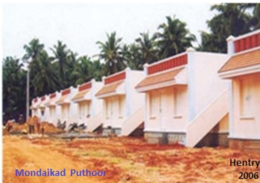
Plate 7. Newly constructed houses at Mondaikad Puthoor
