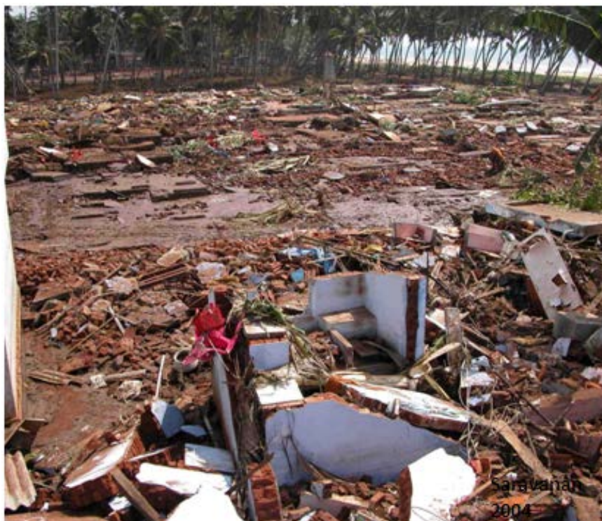
Plate 4. All houses were damaged in Singaravelar Colony
