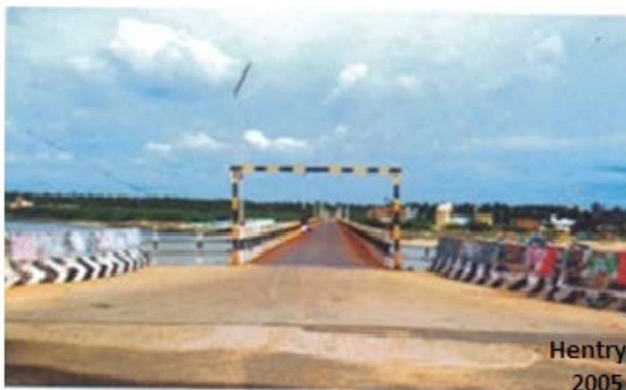
Plate 6. Temporary steel bridge connecting Manakudy and Keezhamanakudy villages
