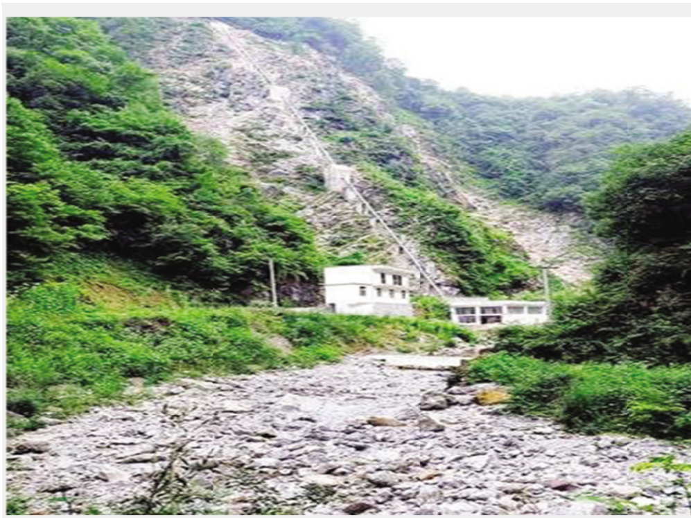
Figure 2. Dried bed of a stream just downstream of the diversion weir of a SHP
