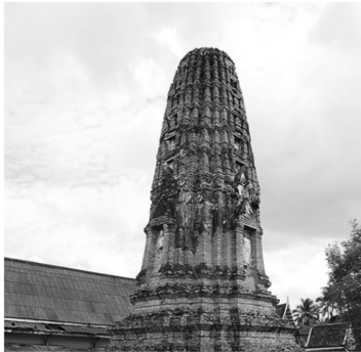
Figure 4. Disrepair of the ruean tat of Pra Prang Luang , Nonthaburi
