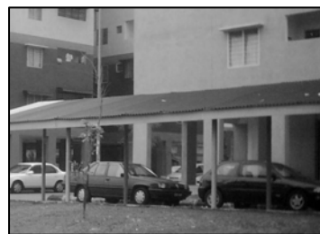
Car parking area
